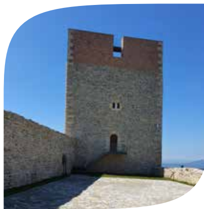
Južna kula nakon uređenja / The South Tower after renovation Izvor / Source: Arhiva JU PPM / Archive of PINPM
